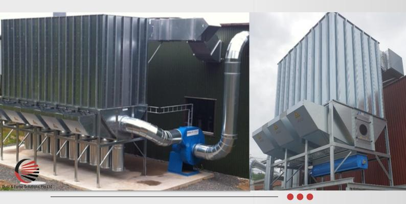
Dust and Fume Solutions has a new range of Filters or Dust Collectors available to give you the Customer the complete range of products to design your new Dust Extraction System. Ranging from Modular Filters through to Super Blower Filters, Dust and Fume Solutions can provide the right Filter for your system.
